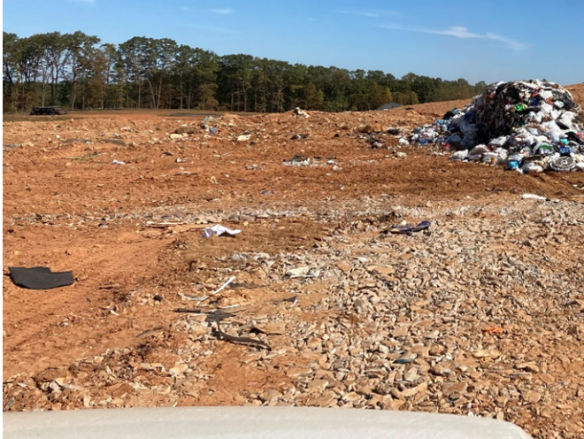
At the time of the inspection, the facility was operating a working face at the eastern area of Phase IV landfill. Some exposed solid waste was observed through the daily soil cover.
