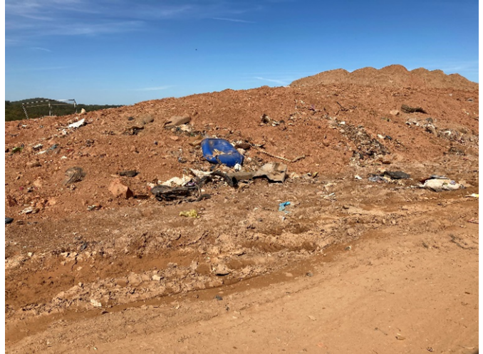
Exposed solid waste was observed in areas under intermediate cover.
