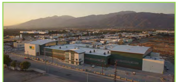
The Azusa Transfer Station and Recycling Facility includes deep foundation elements and a methane gas collection system, a 120,000-sf operating floor, office and maintenance facilities, bale storage, and recycling systems for commercial, single-stream, and green waste.
